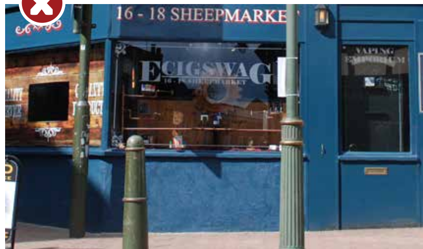
Figure 75: Tall stallrisers reduce the available display space and impact the activity of the frontage.
