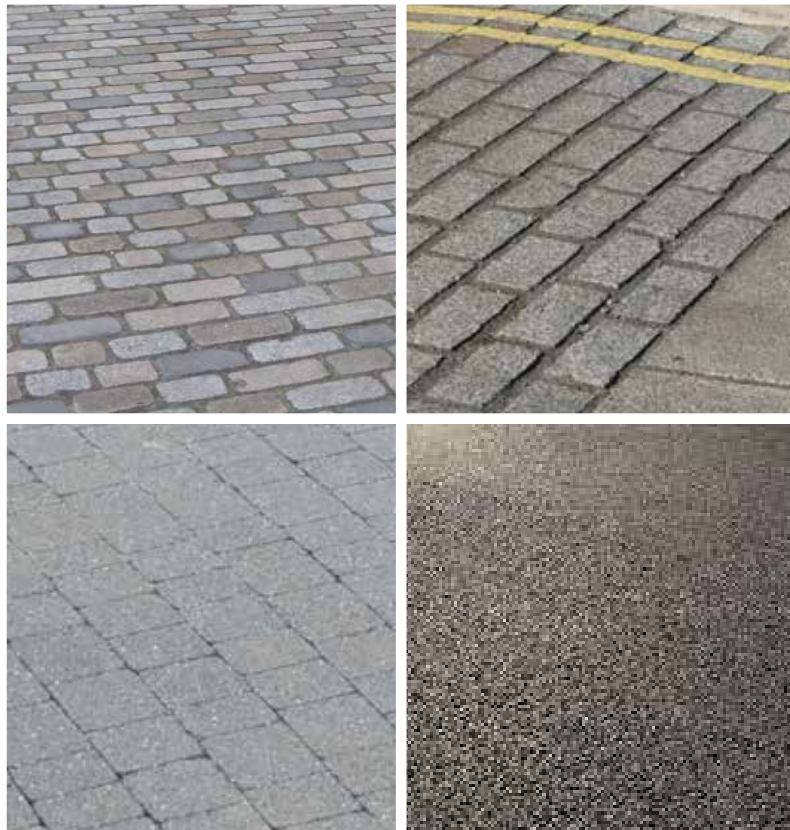
Figure 41: Paving: 1) Yorkstone paving; 2) & 3) Granite paving; 4) Pannat Sandstone. Carriageways: 1) Yorkstone sett; 2) Granite sett; 3) Concrete sett; 4) Asphalt.
