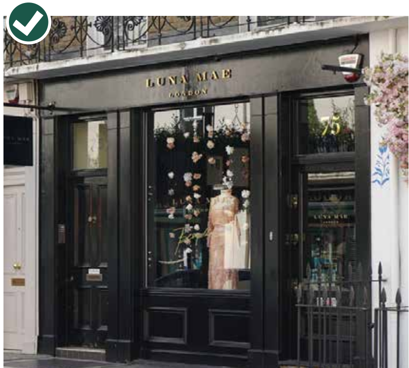
Figure 69: Good example of fascia
