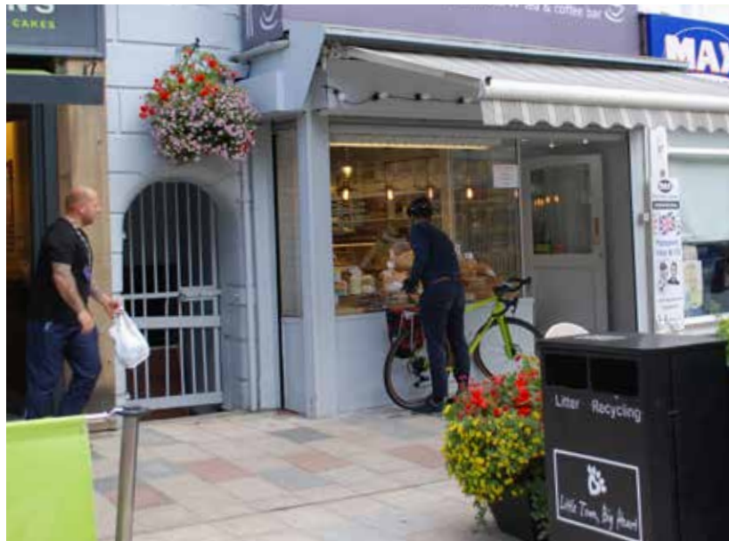
Figure 73: Good example of door and two doorways within one shopfront
