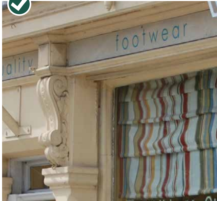
Figure 70: Examples of pilasters
