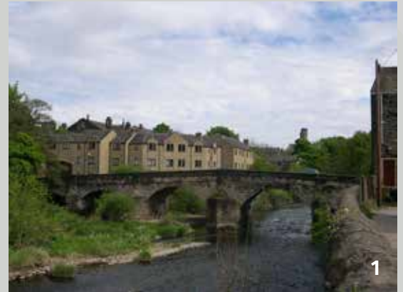
Figure 23: Grade II* listed Ireland Bridge
