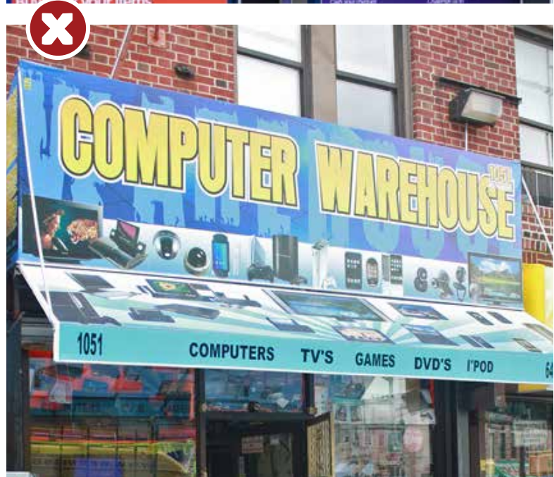
Figure 81: Images above. Bad examples of signage. The designs above, do not have any visual relations with host buildings. The signs contain more than just the business name creating clutter and messy appearance.
