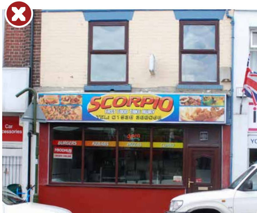
Figure 68: Bad example of fascia
