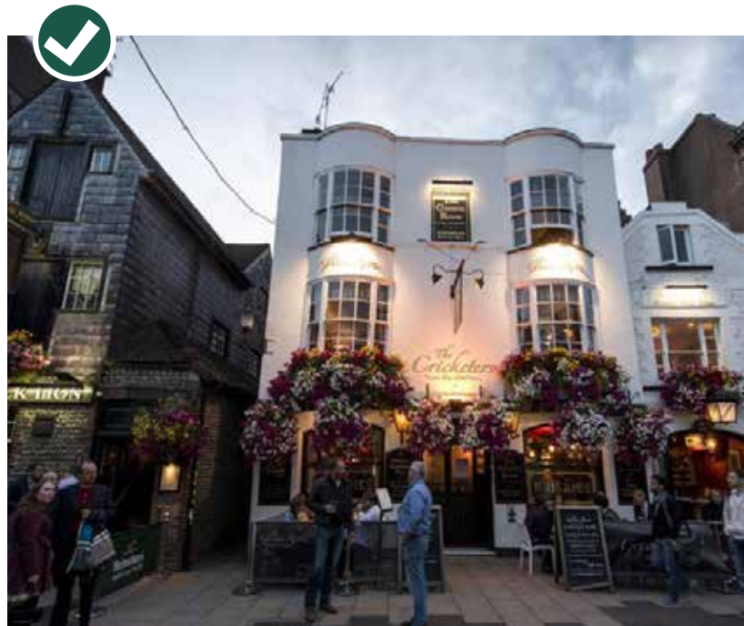
Figure 76: Good example of lighting
