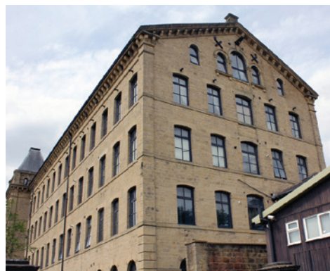
The Locks apartments, Bingley
