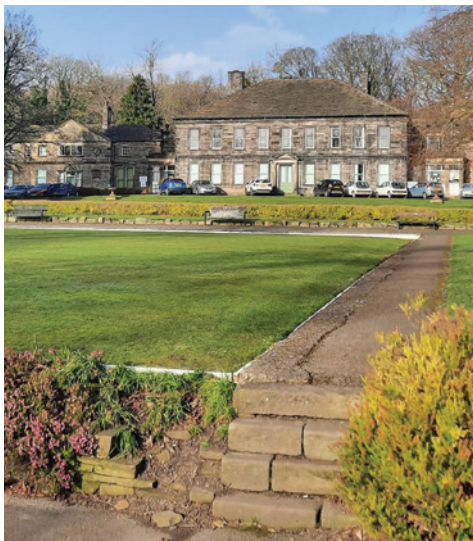
Former Town Hall building, Bingley
